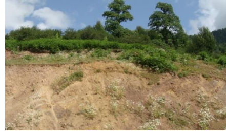
Figure4: Creating a landslide destroyed the
