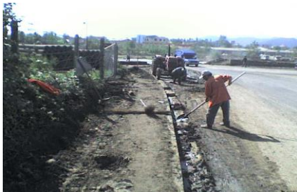
Figure5: The flood destroyed the original
